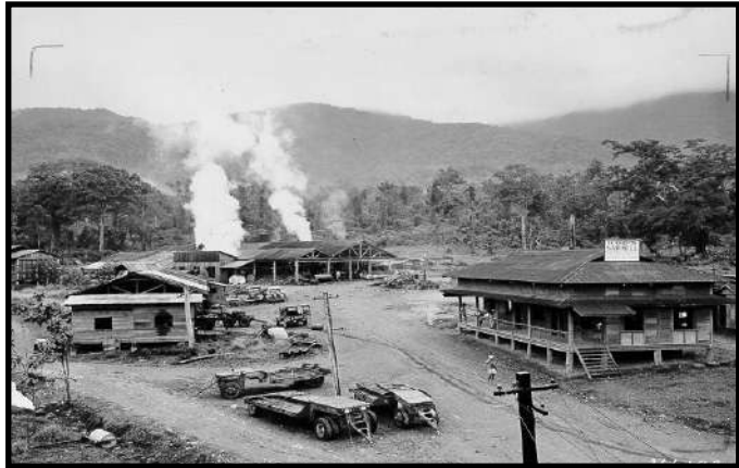
Corps sawmill on Luzon operated by the 1612 th Engineer Forestry Company, April 1945.
